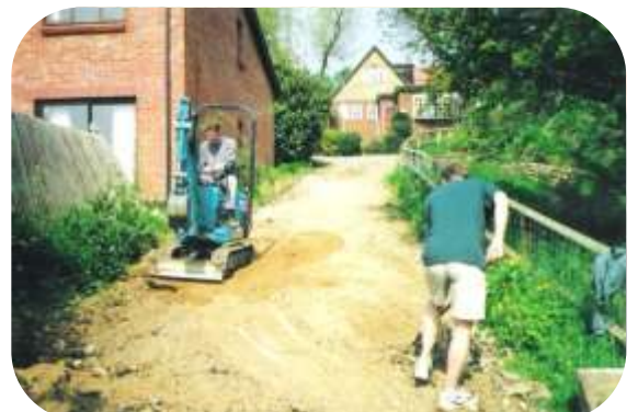
Re-surfacing of the WWA driveway sometime in the last century!
